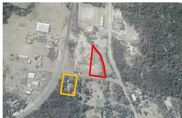
Plate 6: 1986 aerial showing detail of the now cleared OFGS site – same annotation as above (source: NSW Spatial Services with Niche annotation)
